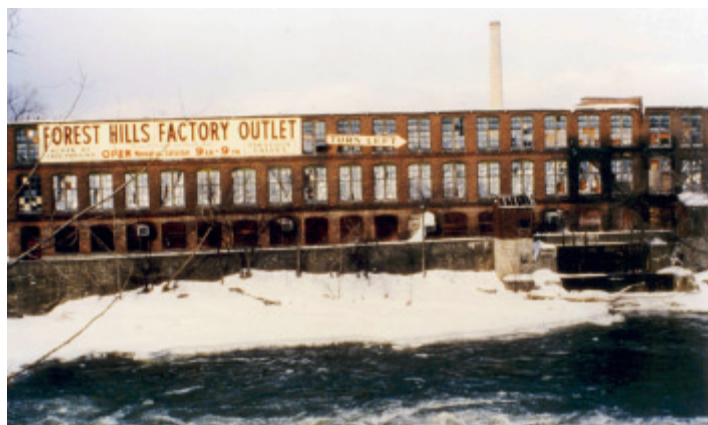
The Woolen Mill 1958 (East Elevation)
