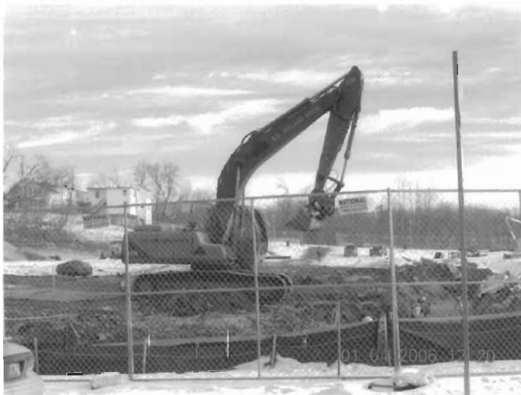
Figure 1: Erosion controls in place at Barlow Place construction site
