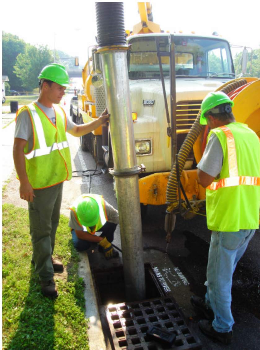
WPCD staff cleaning and stenciling catch basins
